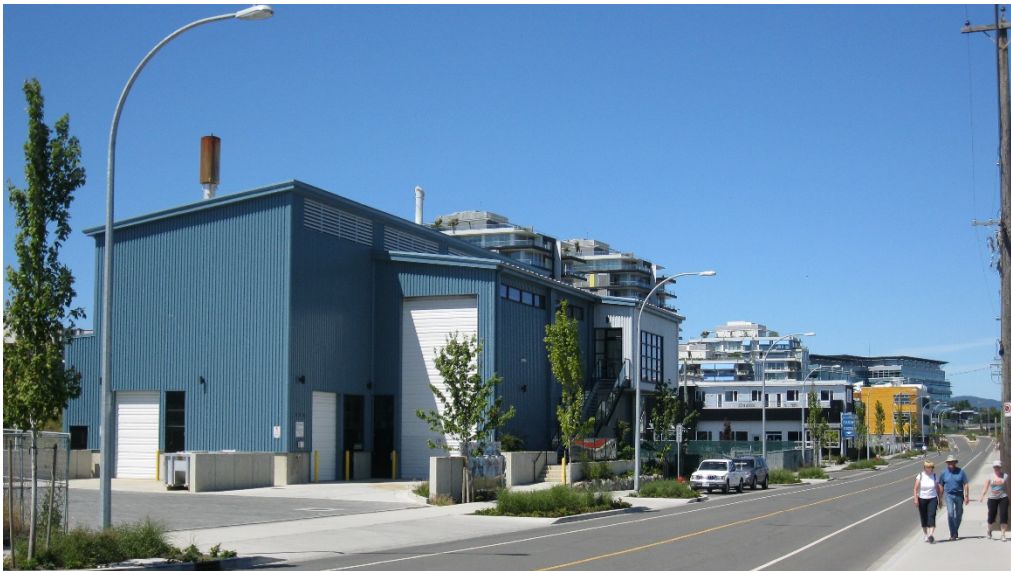
Nextterra Biomass Energy at Dockside Green, Victoria, B.C.
